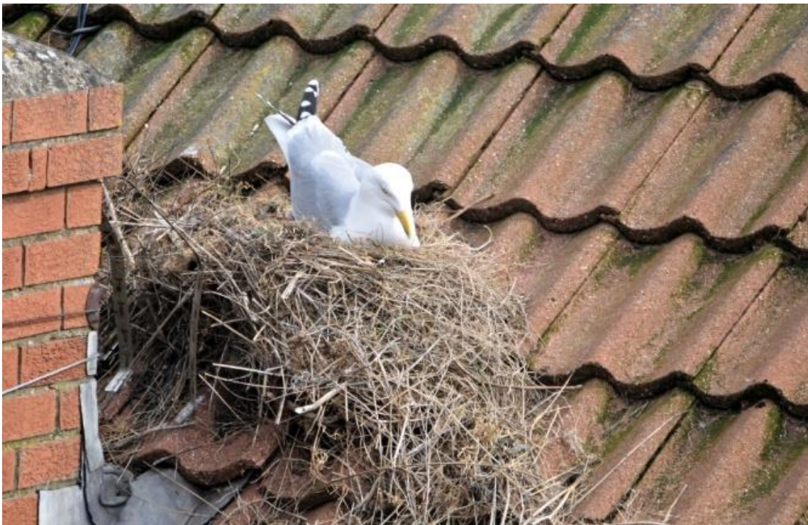
Figure 3: Herring gulls nesting on roofs and between chimneys in urban environments.
